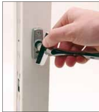
The handle, with the cover plate, is pressed onto the handle plate with the easy snap-in function.
